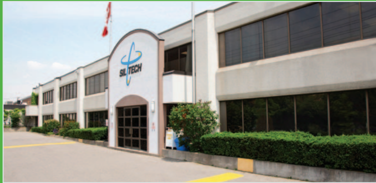
MISSISSAUGA, ONTARIO, CANADA PLANT
